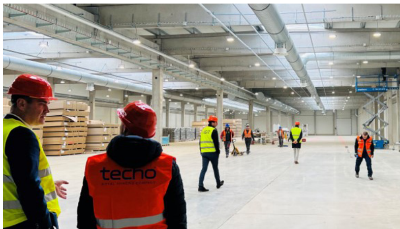
Construction starts on Woodhub Prague, Czech Republic
